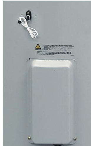
Step 6 remove tape from tank sensor cable
