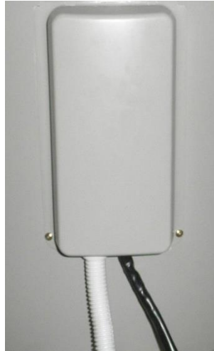
Step 5 refit lower front cover
